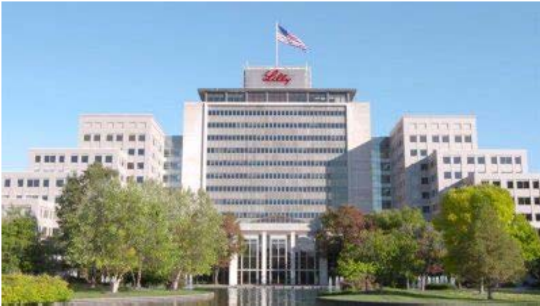
Before Façade Replacement
